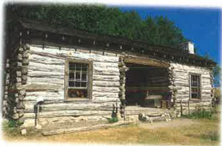
Many of the homes built by early U.S. settlers were dogtrot cabins.
