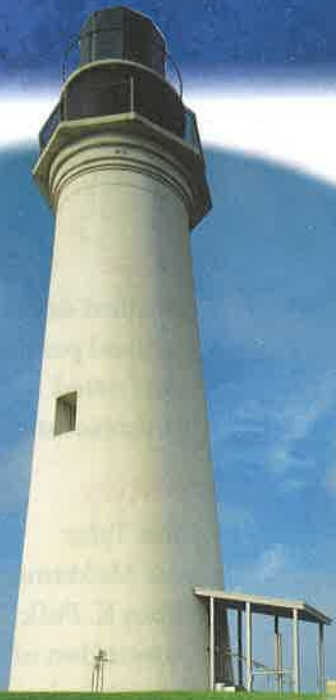
The Port Isabel Lighthouse was used as an observation tower and to signal sailors.
